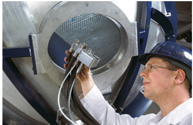
Optimization of Steam Generator primary side cleaning process.
